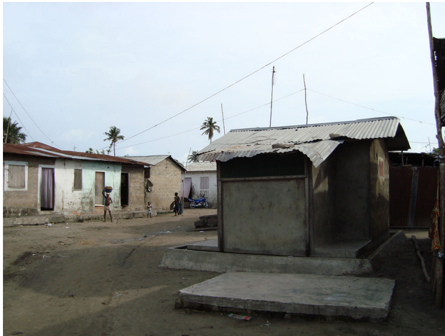
Figure 3 One of the experimental huts (on the right) used for the trial. These huts are located inside Ladji village and houses can be seen on the left
